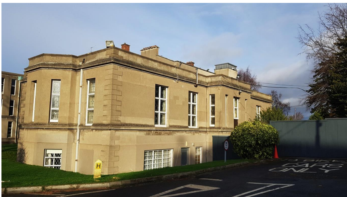
Plate 7.3.21: The front elevation of the Finlay Wing as viewed from the south
