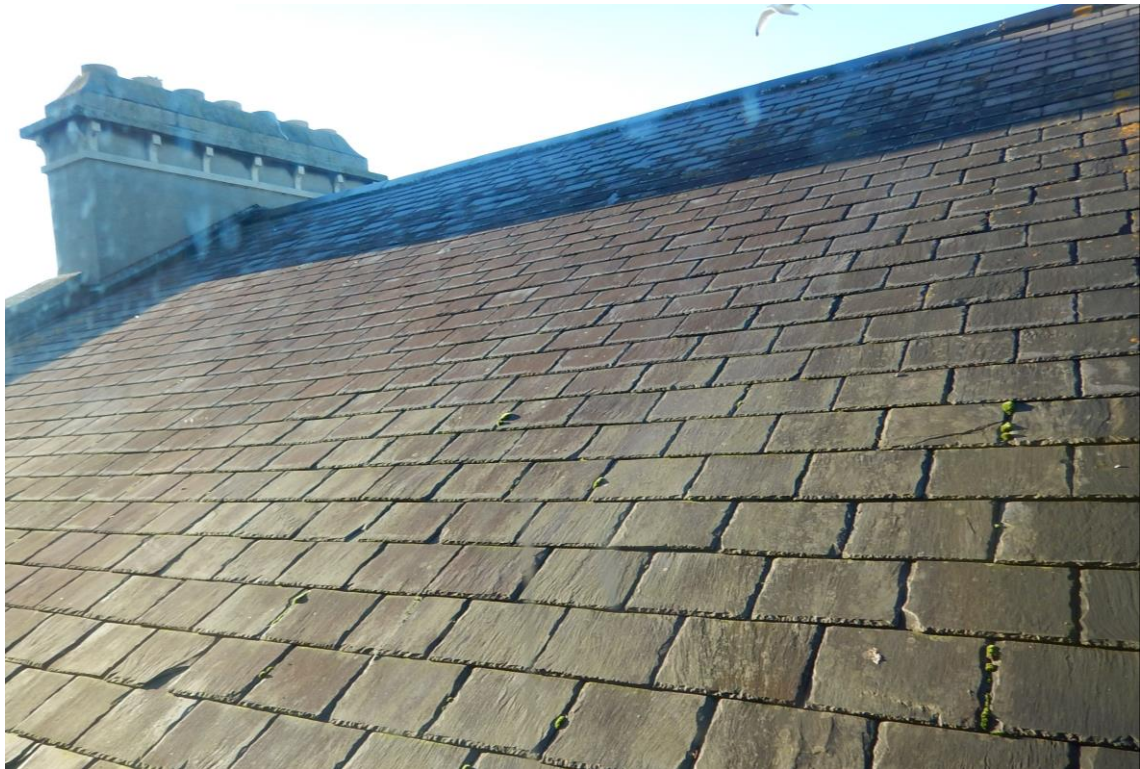
Figure 8.12: View of intact roof at the western end of Milltown Park House.
