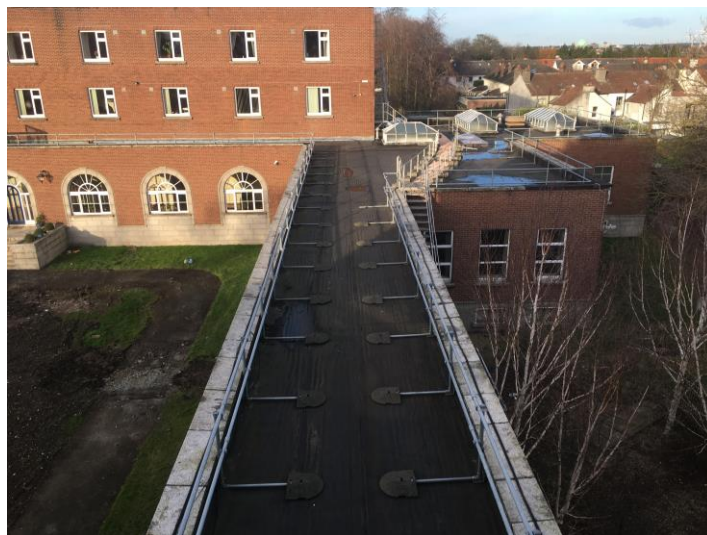
Plate 7.3.20: Flat roof over link building, and its connection with the Jesuit Community Building
