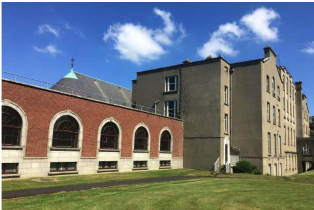
Plate 7.5.1: The red-brick link building (c.1955) connects to the west gable of the rear extension (Building B)
