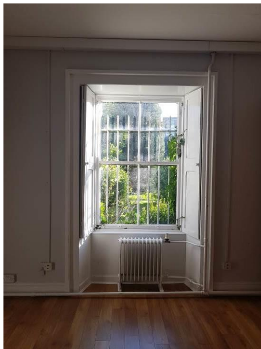
Plate 7.9.2.: The new partition walls are positioned at an appropriate distance from the extant windows to avoid interfering with the composition of the architraves and shutter boxes.
