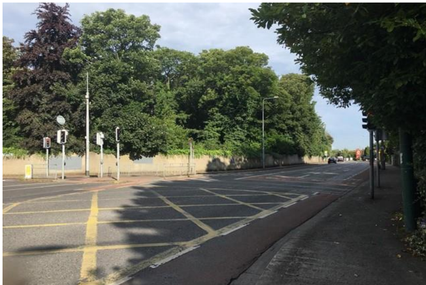
Plate 7.3.6: Sandford Road, due north, from the junction of Clonskeagh and Eglington Roads
