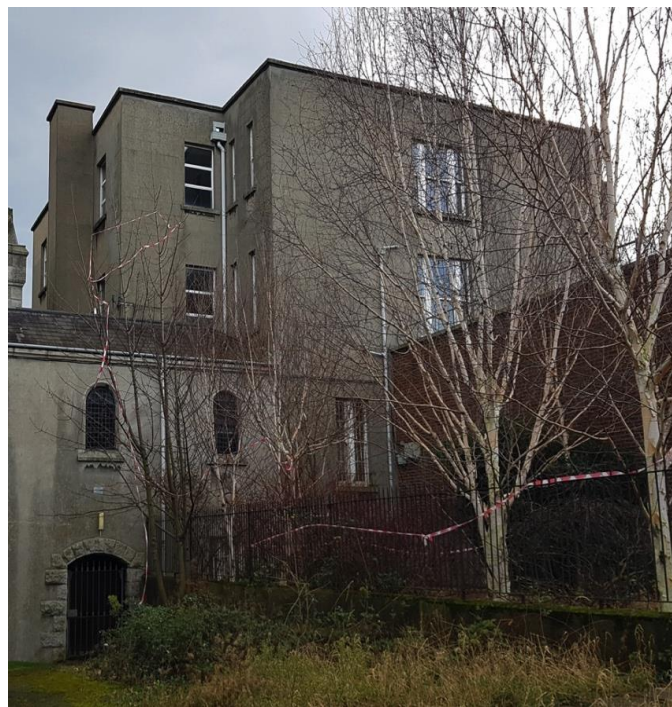
Plate 7.3.18: The rear, west elevation of the rear extension, with two storeys over basement brick link to the Community House, the visible section in this image of which will be demolished as part of the proposed development
