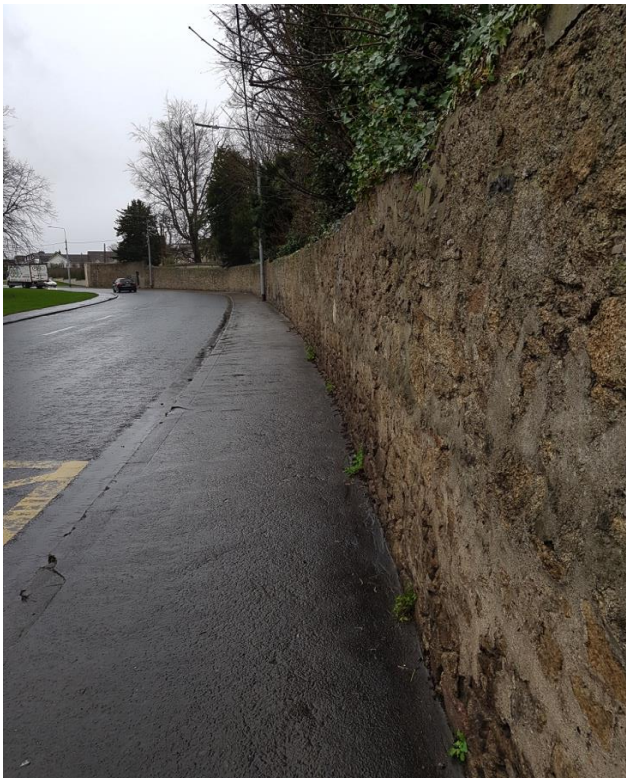
Plate 7.3.31: Boundary wall along Milltown Road
