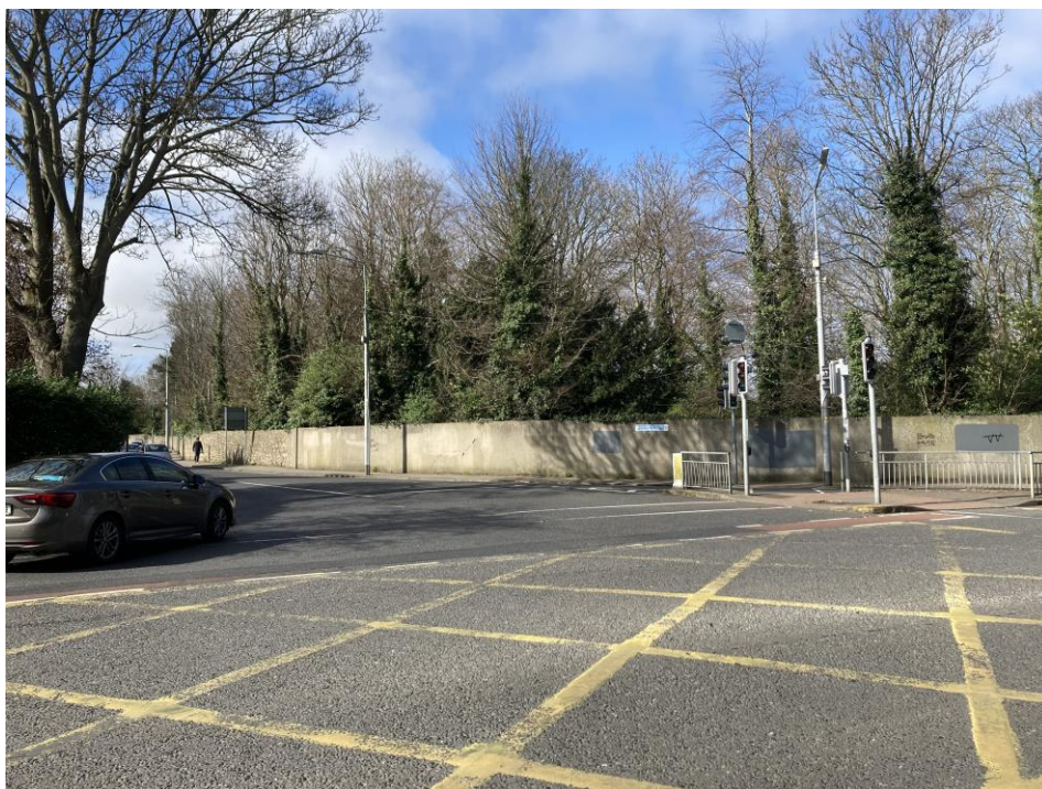
Plate 7.3.32: Replacement section of boundary wall at junction of Milltown and Sandford Roads
